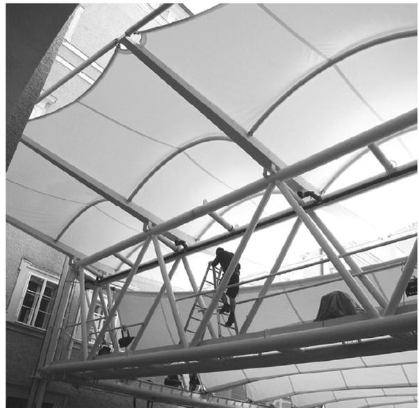
Fig 40: View of the east side shelter protecting the whole membrane when folded. (Courtesy of Kugel Architects).
