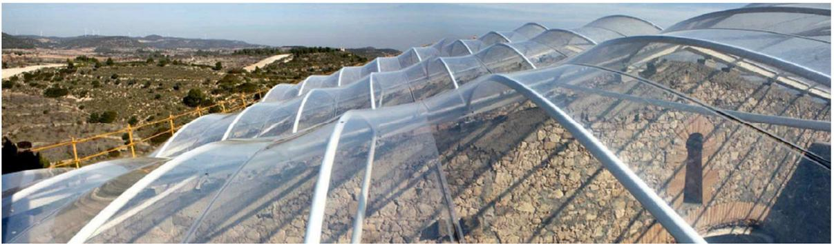
Fig12: Valley cables stretch the membrane and provide double curvature.
