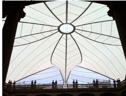
Fig.26: The radial scheme maintains the central symmetry
