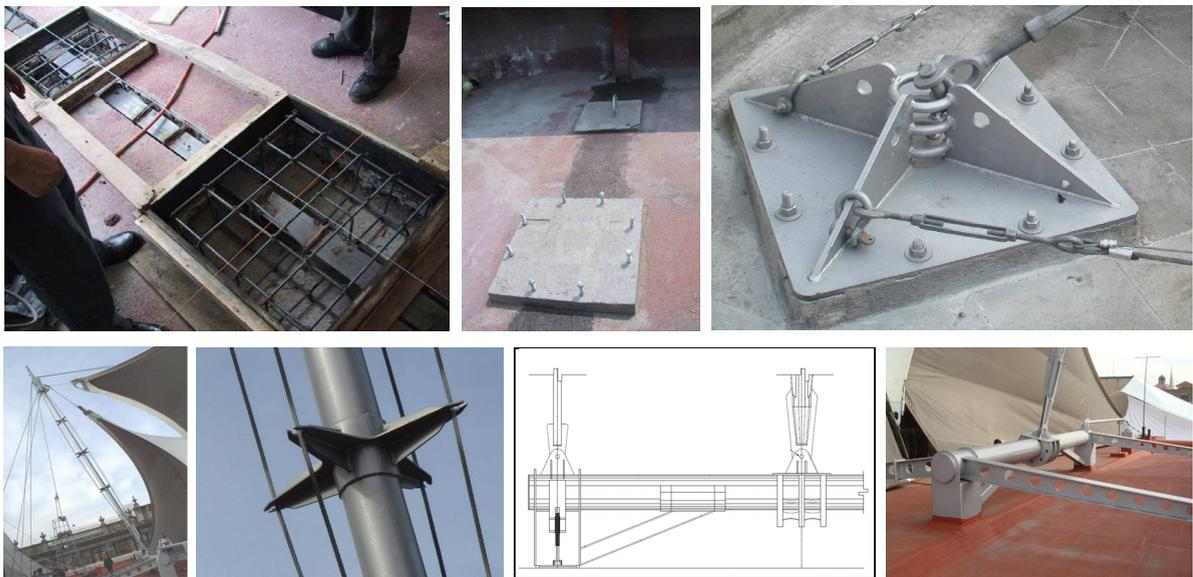
Left to right and top to bottom: Figs.18, 19, 20: Plates anchored in the concrete slab pored during a previous restoration. Figs.21, 22: Prestressed masts. Figs.23, 24: Masts are pinned on CHS acting as beams between plates.
