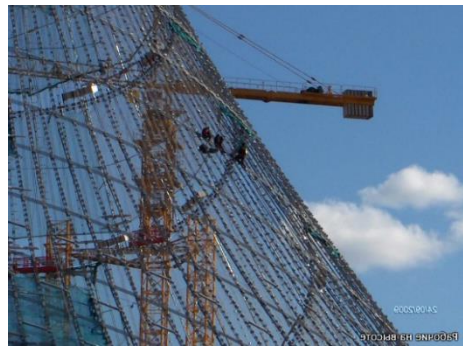
Figure 17: Khan Shatyr in Astana and cable net
