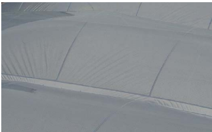
Figure 20, Too much distortion in the cutting pattern causes wrinkles in the cushions
