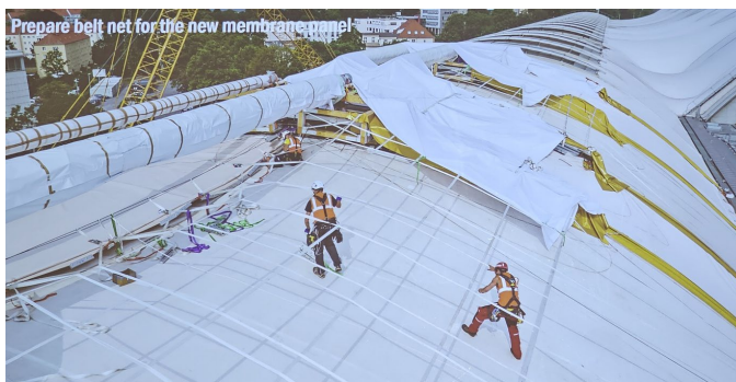
Figure 1. Renovation of Dresden Central Station Membrane Roof © Pfeifer Structures
