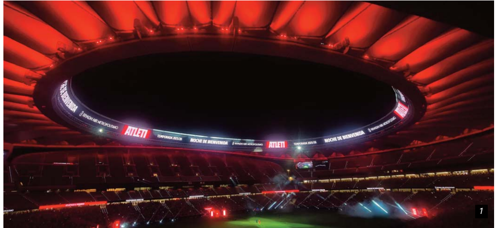
Figure 1. The sky ribbon installed between the upper and lower tension rings of its bicycle-wheel-shaped roof.
