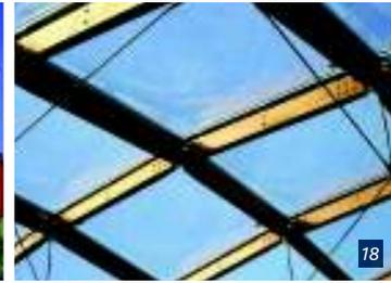
this envelope is the printing of the fabric that needs to be related to the cutting patterning in order to maintain the design. The renovation of the old Arena was also based on wrapping the building with decorative panels, thus demonstrating, together with the new one, that textile façades are a new growing market for fabric architecture.
