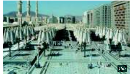
Figure 15a-b. Foldable umbrellas of the external courts of the Medina Haram Piazza
