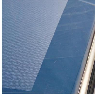
Figure 2b: Details of stable print pattern, after 23 years installation on the roof of the atrium (2015)
