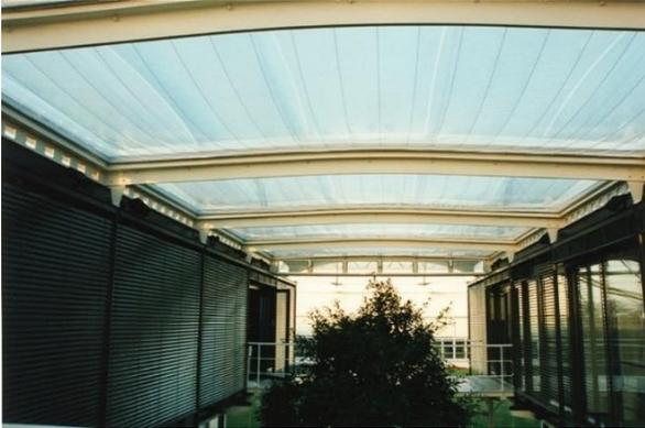
Figure 2a: ETFE atrium roof Schlumberger Research Institute, Cambridge, UK, outer foil printed on inner surface, print pattern DM 4:65, light optical density ink (1992)
