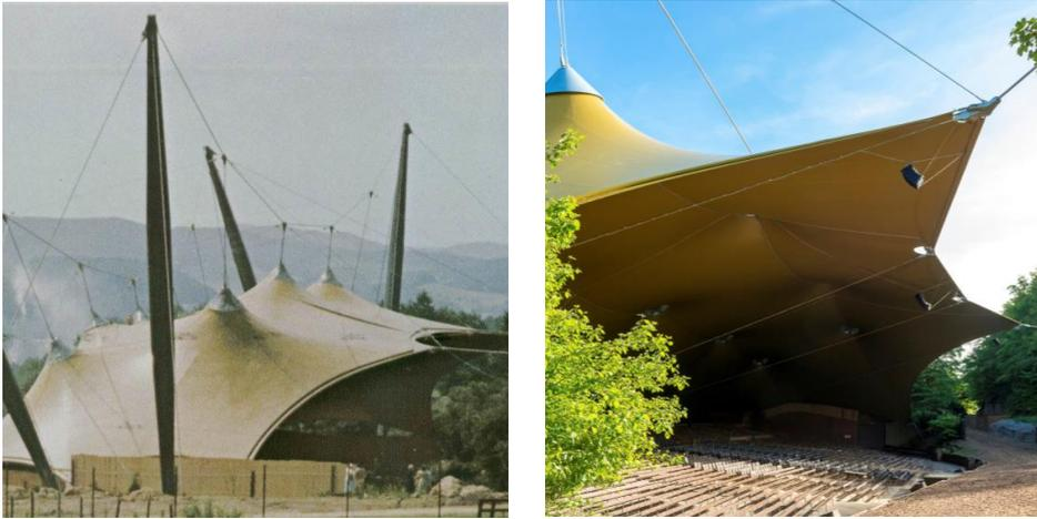
Figures 1 and 2: Elspe, Grandstand Canopy, Figure 1 shows the original project from 1978 © Mehler Technologies, figure 2 shows the replacement from 2015 © Koch Membranen
