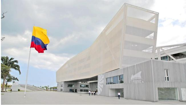
Figure 4: office building in Ecuador with a textile wrap, TF 400
