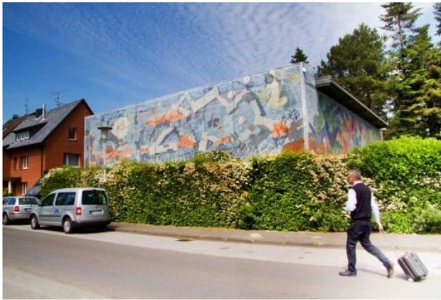
Figure 8: textile mesh façade for a one family house , printed TF400
