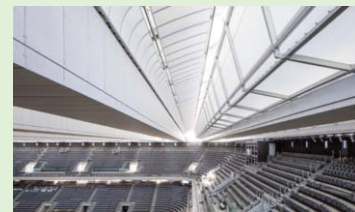
Retractable roof Philippe Chatrier © DVVD Architectes
