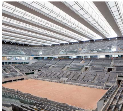
Retractable roof Philippe Chatrier © DVVD Architectes
