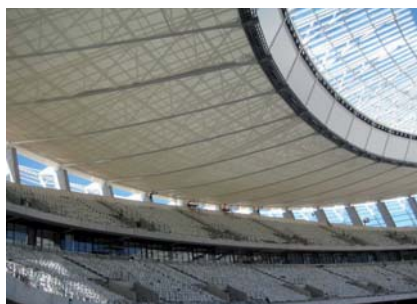
Fig. 2 Detail of wave-shaved roof of the Cape Town Stadium.
