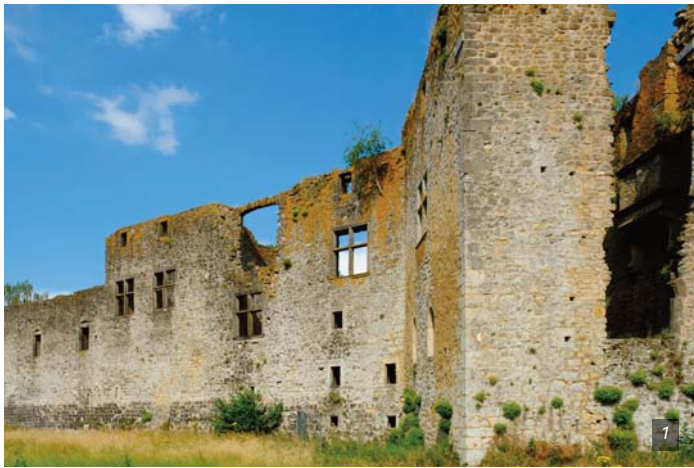
Figure 1. The Koerich Castle, the situation before the intervention in 2018 © Ney & Partners
