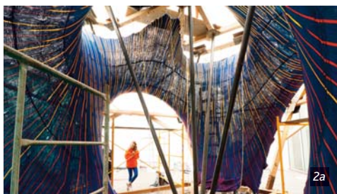
Figure 2a. Cable-net and knit formwork tensioned in between the external frame © Maria Verhulst
