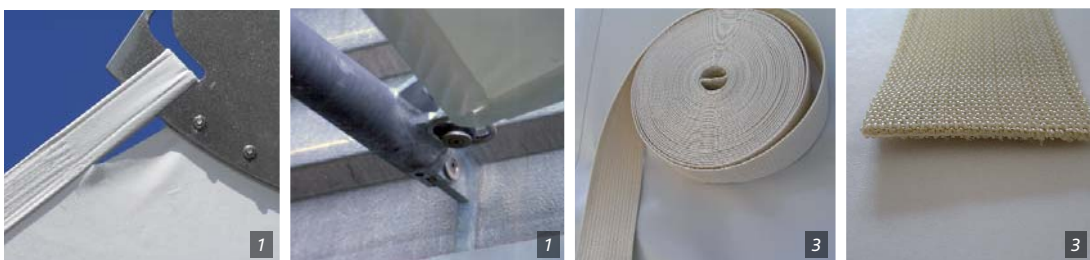
Figure 1. Edge detail with a belt in a sewed pocket
