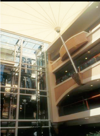
Fig. 2.13 Non-uniform prestress field
