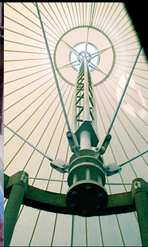
Fig. 2.29 Jacked flying mast
