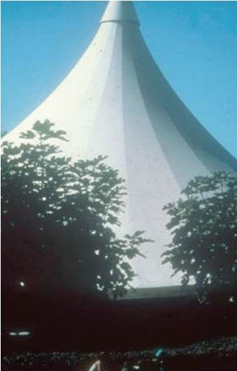
Fig. 2.12 Radial cables lying in contact with membrane's surface
