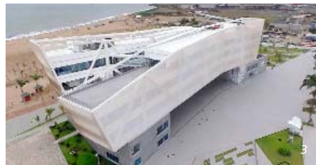
Figure 1: Dar Al-Handasah Consultants with Maffeis Engineering SpA, Taiyo Middle East and Pfeifer, 2014: Khalifa International Stadium, Doha.
