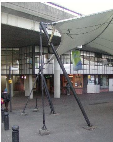
This is the simplest case. The foundation is subject to the vertical pulling load  $F_y$ . To provide stability, the foundation will resist this force in several ways:
