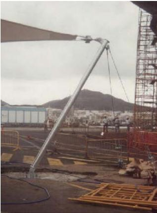
Inclined compression force is a very common case in tensile constructions. In fact, it is usually more common than vertical compression. Inclined masts are used, above all, to increase the lever arm of the moment that form the vertical reactions at the base of the masts and the stay cables, in most of the perimeter supports (bipods or tripods) .
