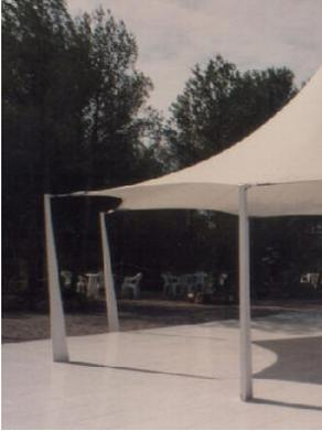
In some cases, especially in the perimeter of tensile constructions we find solutions based on bipods (a mast and a stay cable) or tripods (one or two masts with two or one stay cables respectively) and even more complex sets of masts and stay cables.
