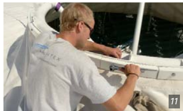
Figure 9. Roof top view Figure 10. Different stages of high point installation Figure 11. Installation of the high point clamping profile
