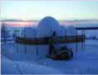
Figure 1 A two-storey snow hotel covered with the snow (reception in the centre, 8 rooms around)
