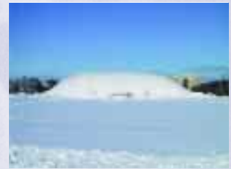
Figure 3 Airhall of 100m x 60m x 18m
