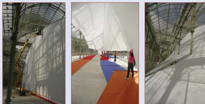
Figure 4. The membrane attached to the arch
