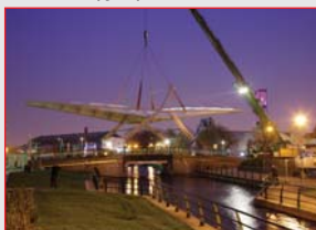
Canopy Structure lifted into place
