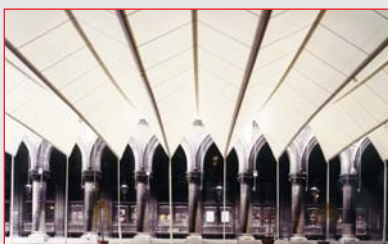
Fig. 10. Mobile spectator stand, using a scissor structure to support a membrane
