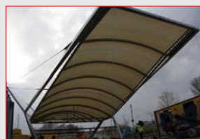
Fabric Canopy in place on Frame
