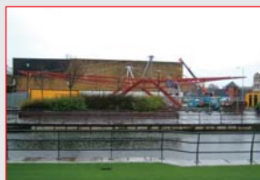
Steel Frame on the Canal side
